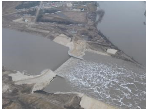
Floodway outflow north of the Lockport Dam Province of Manitoba photo
