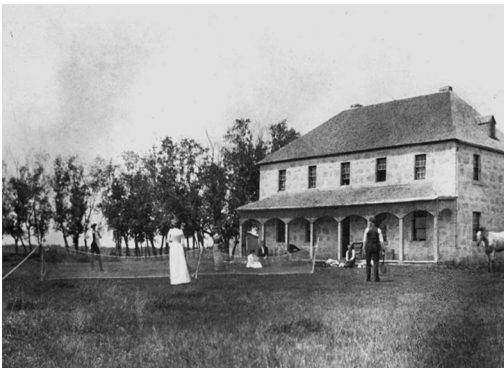
St Andrews Rectory c. 1906
