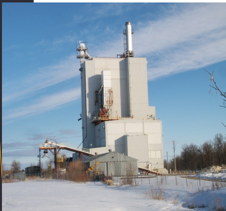
Dow Corning plant
